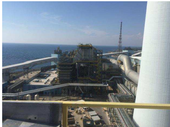
Side view of a tubular flue gas cooler.
